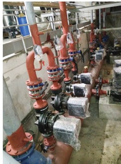
Works on the main heat exchange station
