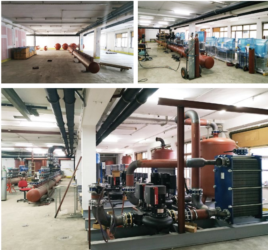
Works on the reconstruction of the main cooling station
